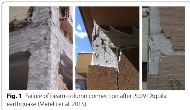
**Fig. 1** Failure of beam-column connection after 2009 L'Aquila earthquake (Metelli et al. 2015).
