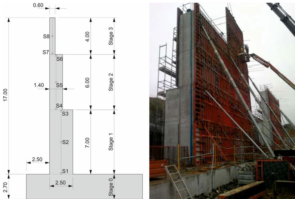
**Fig. 15** Retaining wall construction in Loja (Granada, Spain): **a** main dimensions of the wall in meters, location of the temperature sensors S1 to S8 and indication of the construction stages and, **b** in situ construction of the wall.
