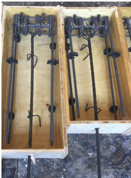
Fig. 2 Specimen's preparation before concrete casting
