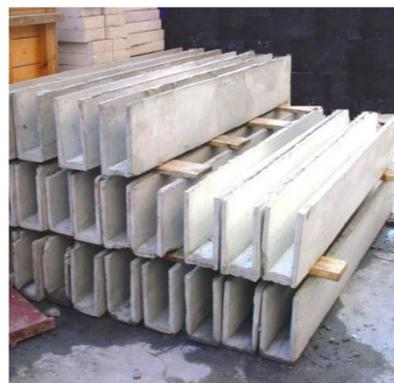
**(d)** The U-shaped ferrocement forms
