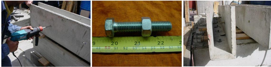
(a) Drilling the holes for the connectors (b) Mechanical shear connectors (c) Mechanical shear connectors arrangement
