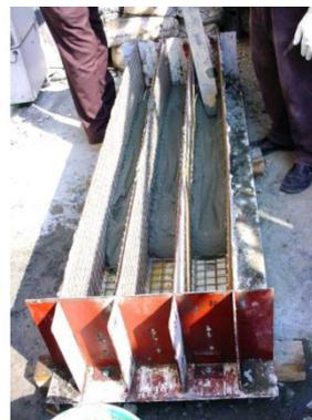
**(b)** Casting the bottom of the U-shaped forms
